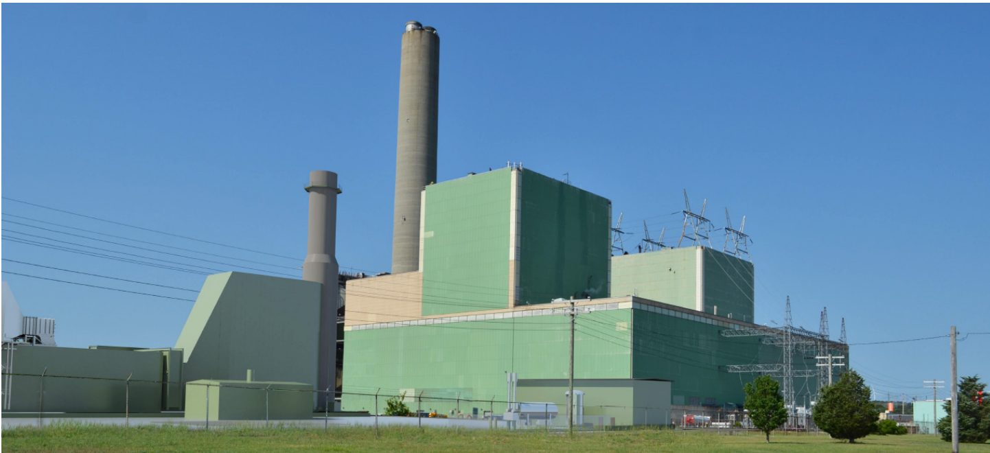
Canal Generating Station, Sandwich, Massachusetts
